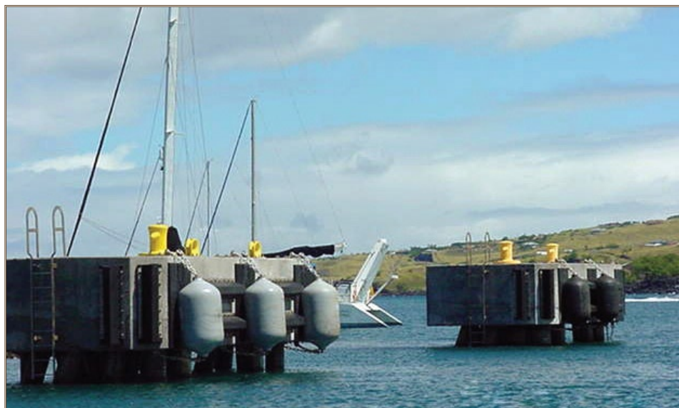
Dolphins in the Kawaihae Harbor are being used to study a composite wrap’s effectiveness in protecting against corrosion. Photo courtesy of USAG Hawaii
