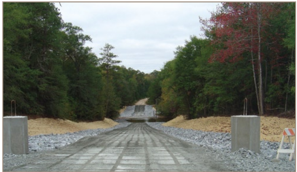
The low-water crossing sites were remediated with articulated concrete slabs, constructed with cable concrete, which allows for movement of the track vehicle. The cable concrete is placed underwater on the river bed to minimize the disturbance caused by the tank. Entrance and exit slopes are also hardened reducing suspended solids released into the waterway.
