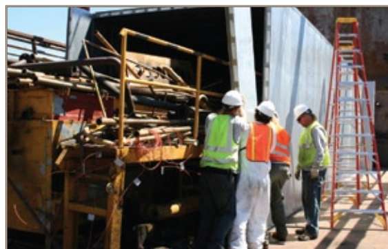
Workers build an insulated enclosure around TNT washout facility equipment at Tooele Army Depot, Utah. The FRP project employed, thermal convection to bring down an unwanted ammunition facility. Photo by Debra Valine
