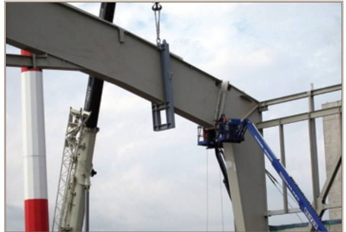
A structural steel installer at the $22 million Ramstein Air Base C-130 hangar bolts together sections of the 355-foot main beam. Photo by James Wofford, Europe District project engineer
