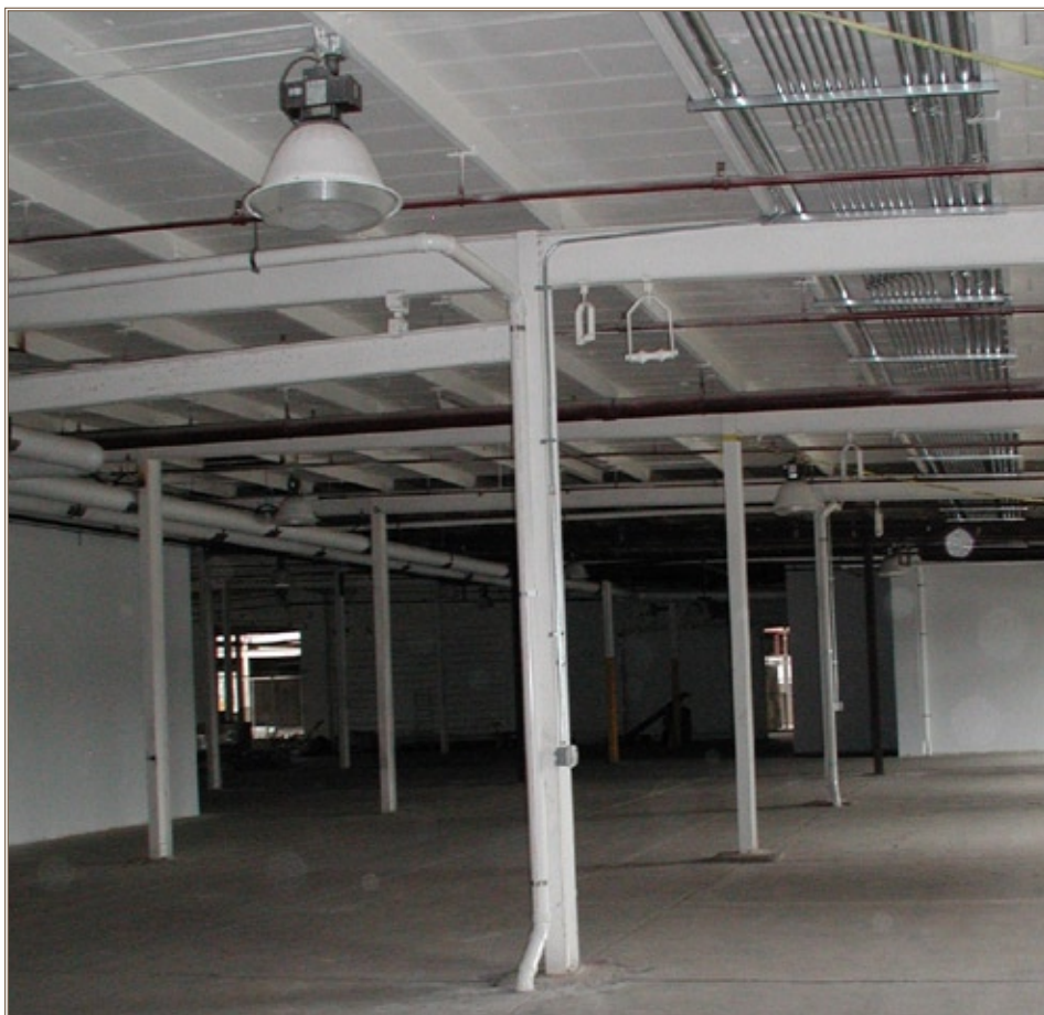
Pipes installed in floor slabs allow contaminated soil vapors to be drawn into a piping system and escape to the outside of a building. Photo by Mark J. Fisher
