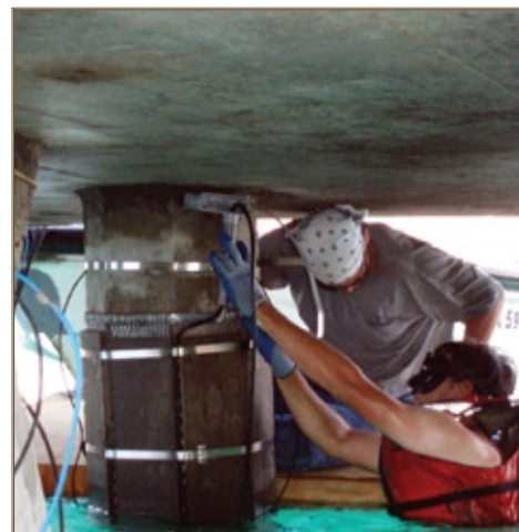
Divers install a composite wrap, a mesh material that provides cathodic protection, on dolphins at Kawaihae Harbor. Photo courtesy of CERL
