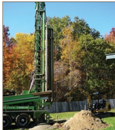
This drill rig will be used to install the ground source heat pump at Londonderry AMSA. Photo courtesy of Alares LLC
