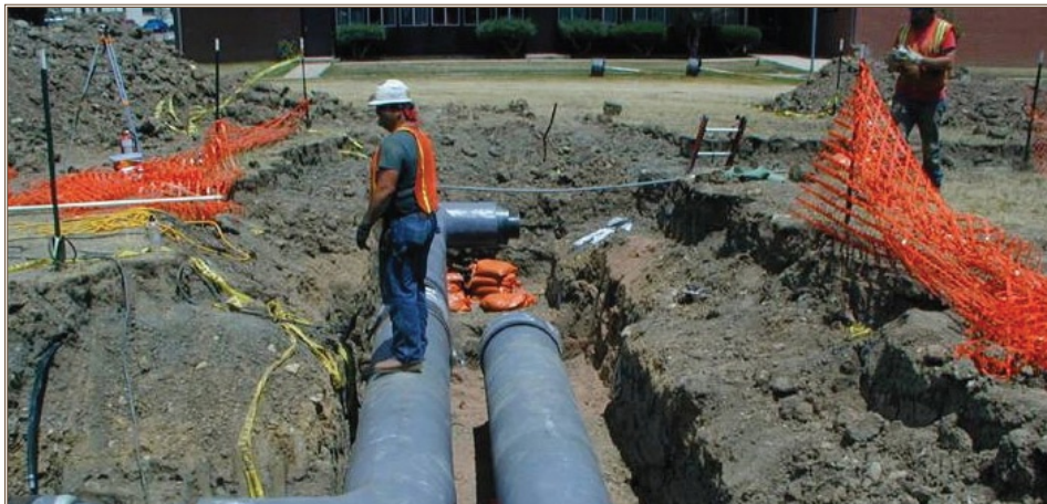
High-density polyurethane- and FRP-clad heat distribution pipes are being analyzed after three to four years in service. Photo courtesy of ERDC-CERL
